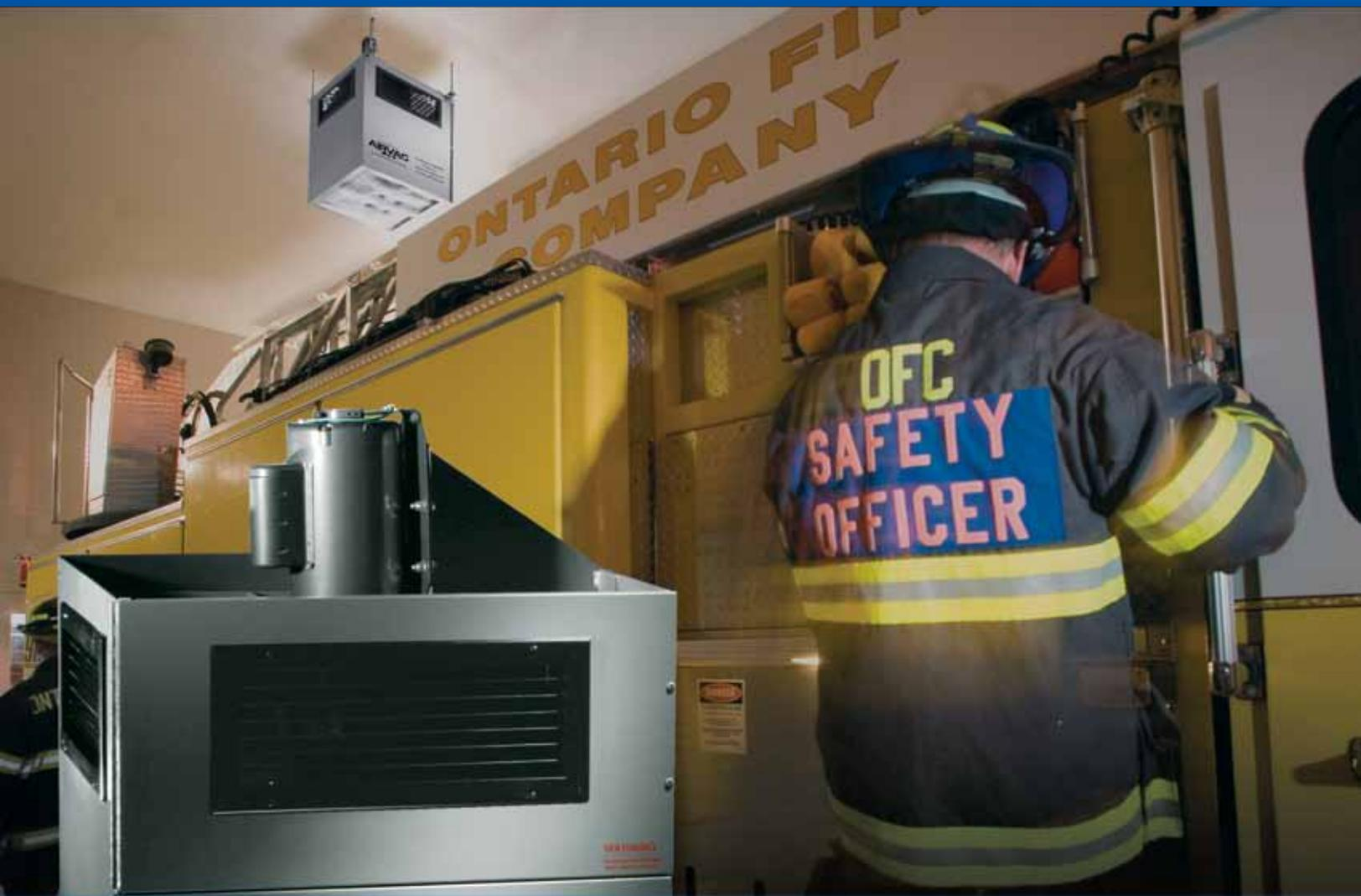
**AIRVAC 911<sup>®</sup> Engine Exhaust Removal System**
